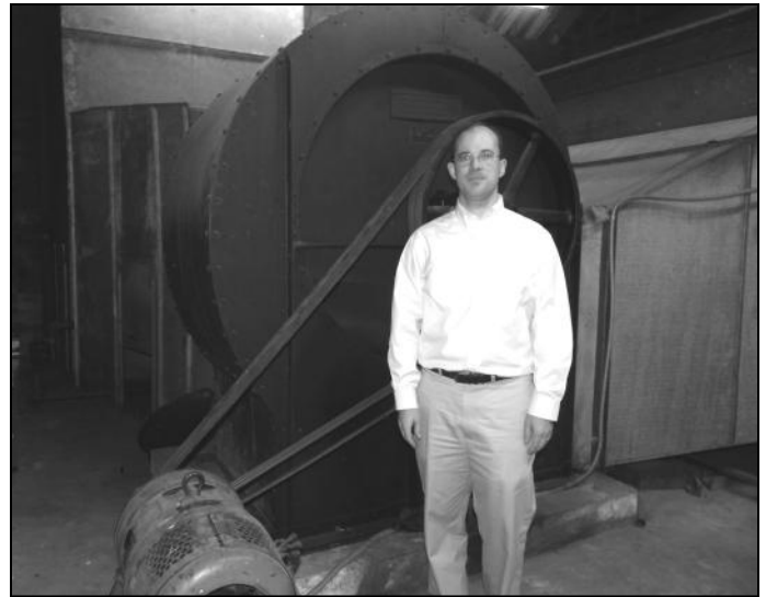
Board President Ray Kahler in front of the original blower which is located in the attic above the projection booth. This blower will be incorporated into the new system.
