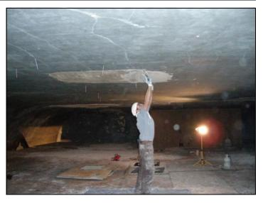
Nick from EverGreene plastering the ceiling. Note the straws hanging down from the ceiling, marking the star holes.
