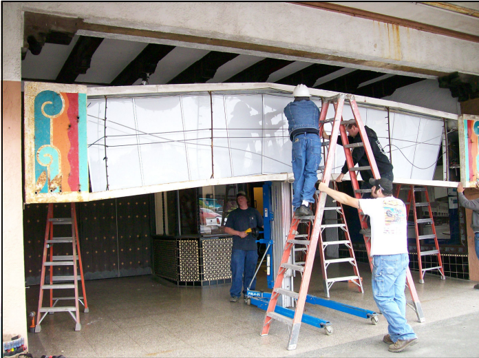
Workers from Phoenix Sign Co. remove the old marquee
