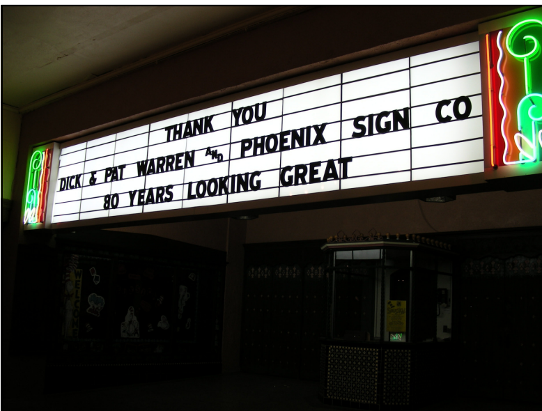
The new marquee is a replicate of the original, incorporating the original tracking system and letters, which have been repainted.
