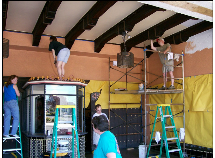
Volunteers paint the entryway on June 28
