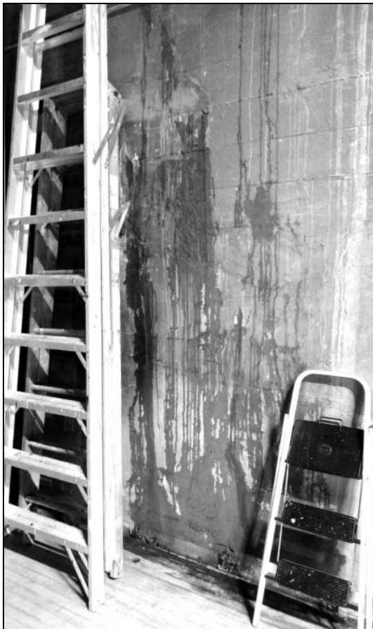
The above photos were taken recently of the back wall water penetration after a rain storm. This is the wall directly behind the stage. There is also water penetrating on the alley side of the interior wall. Containers are placed to capture water.
