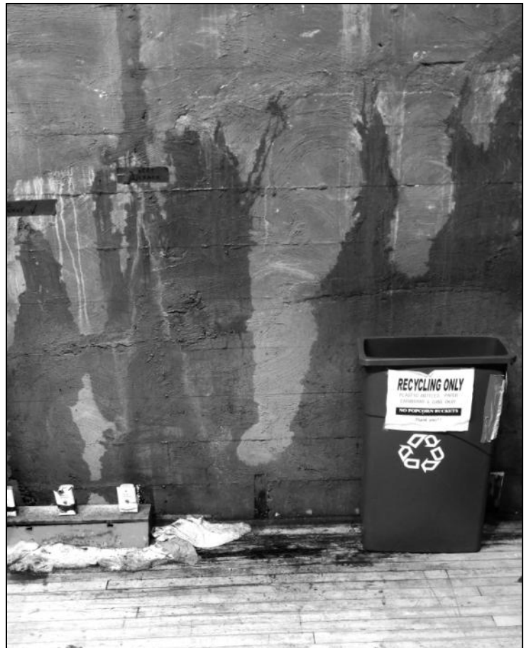
The above photos were taken recently of the back wall water penetration after a rain storm. This is the wall directly behind the stage. There is also water penetrating on the alley side of the interior wall. Containers are placed to capture water.
